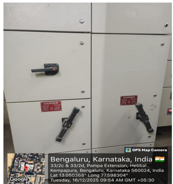
Main Power Supply Board
