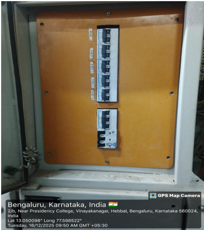
Miniature Circuit Breaker – Floors 1, 2 and Computer Labs
